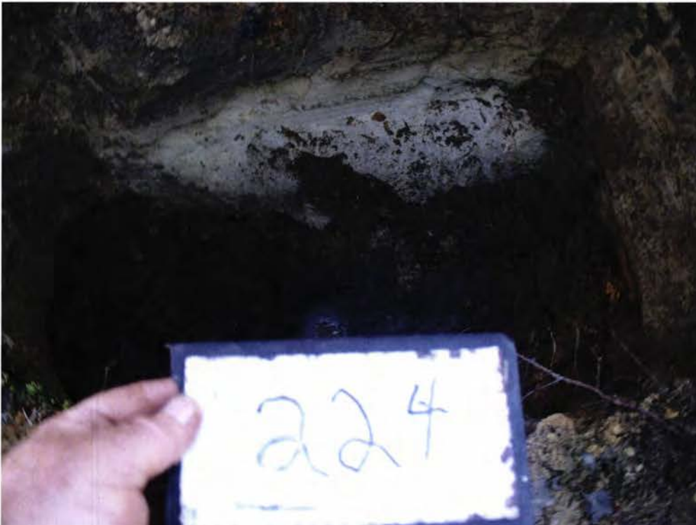
Picture 2: UST 224Cypress tank pit.
